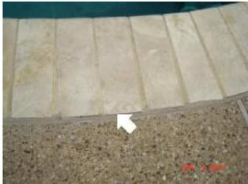
Minor cracks in Deck-O-Seal.
