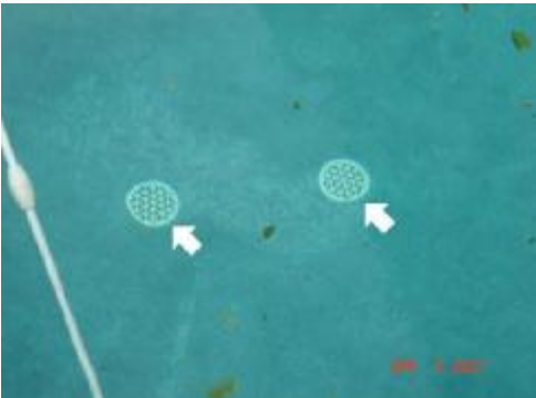
No anti-vortex drain covers.
